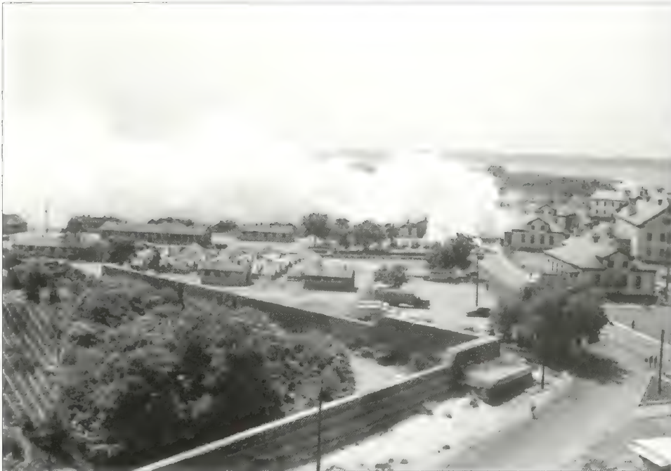
Figure 2.72. View looking southeast at the Mortar Battery, 1943. During World War II, the battery received an upgraded concealment treatment to better disguise the open, concrete mortar pits when viewed from above. Netting with camouflage patterning is visible over the gallery and the southwest mortar pit (GATE 1943-662).
